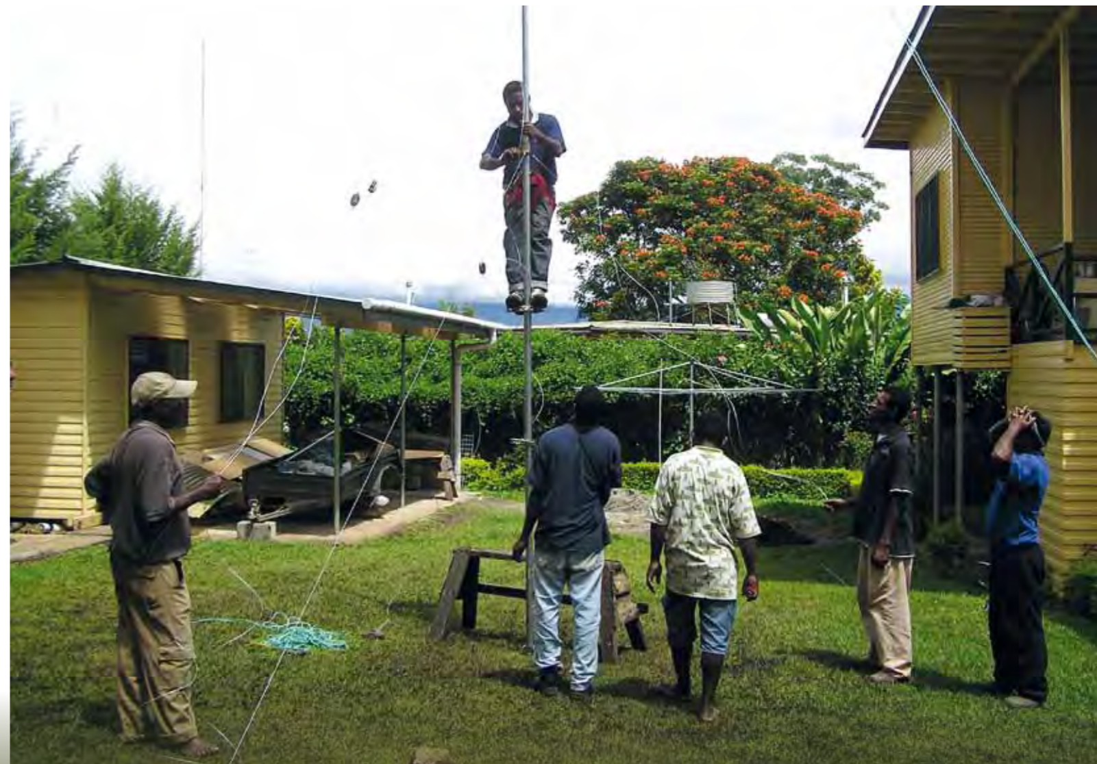
Practical training in erecting an antenna...
